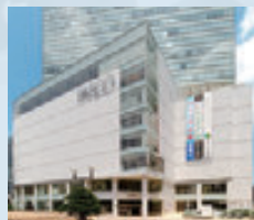
Sendai PARCO, first complex in Tohoku area (Aug. 2008)
