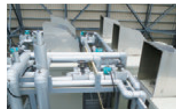
Grey water facilities for purifying rainwater, miscellaneous wastewater and kitchen wastewater
