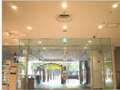
P'es Lighting installation of PARCO SPACE SYSTEMS CO., LTD.
