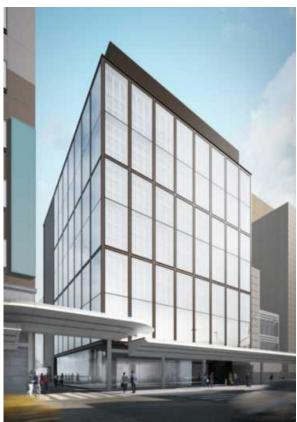
By using ceramic printing on large glass panels, the exterior design evokes the motif of traditional Japanese paper doors. The façade was designed to meet the dignified appearance of the Kyoto townscape.
