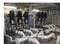
Grey water facility
