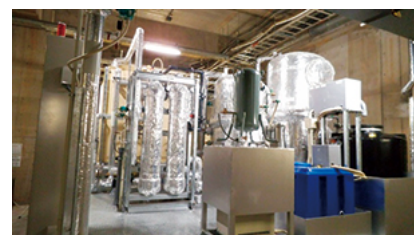
Groundwater filtration system at Nagoya PARCO
