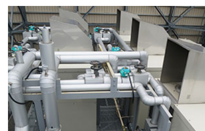
Grey water facility
