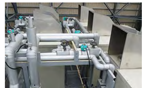
Grey water facility
